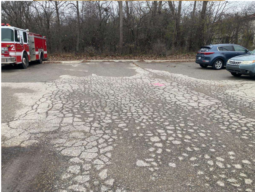
Core Photograph of PC-8: Portland Cement Concrete = 3-3/4 inches
