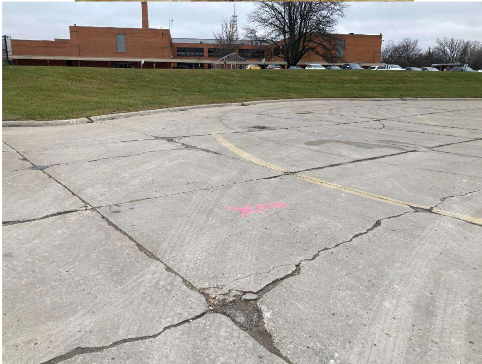
Core Photograph of PC-2: Portland Cement Concrete = 11 inches
