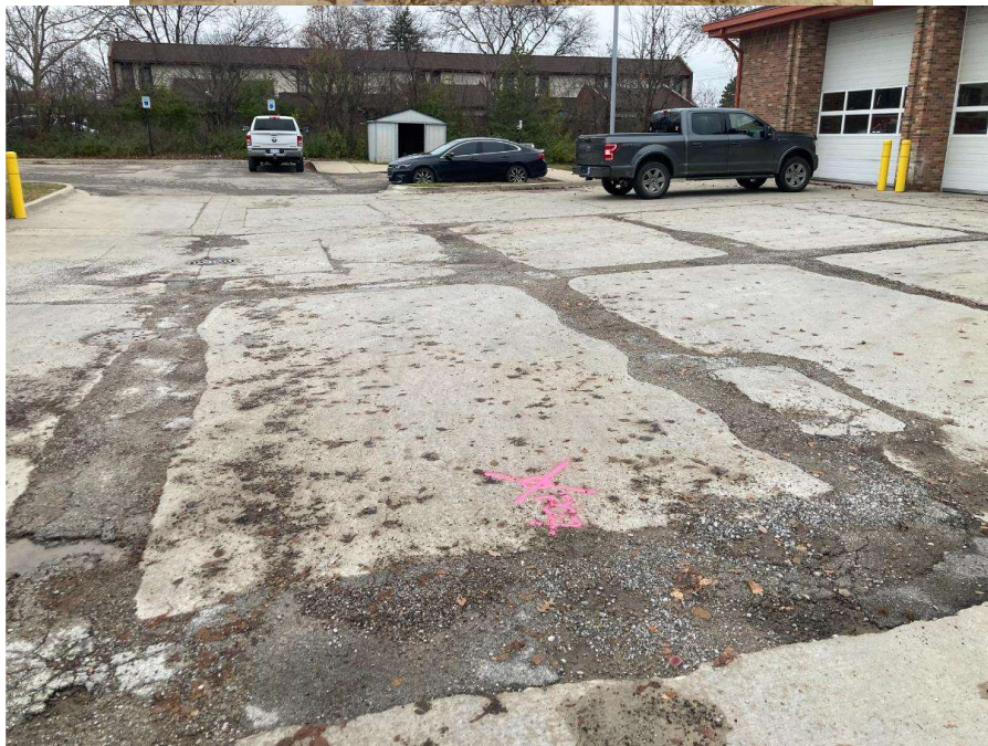
Core Photograph of PC-7: Portland Cement Concrete = 10 inches
