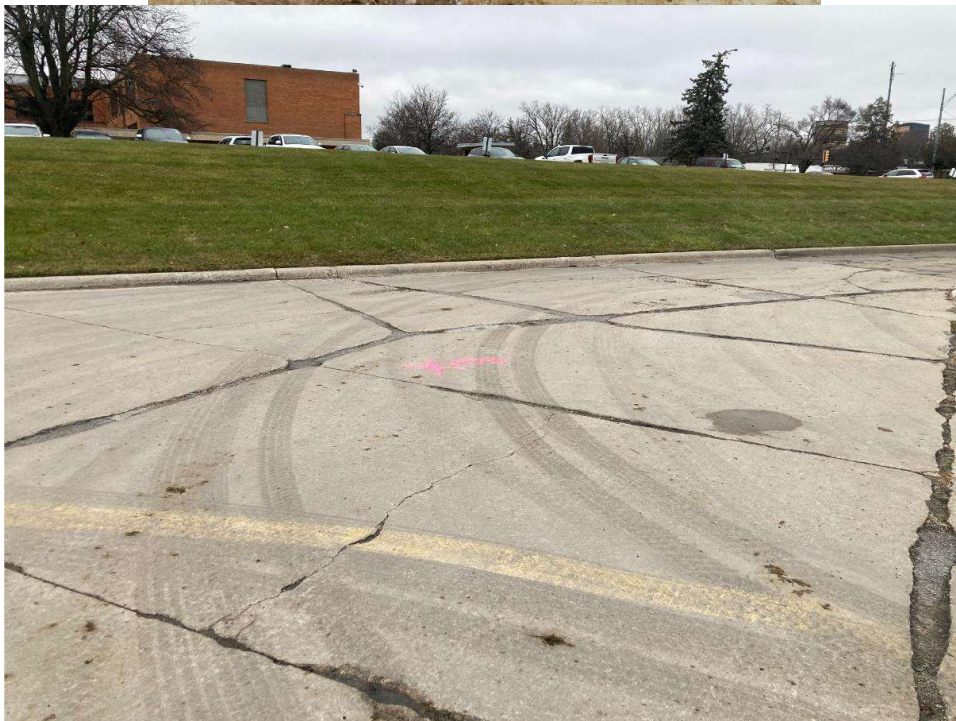
Core Photograph of PC-3: Portland Cement Concrete = 10-1/2 inches
