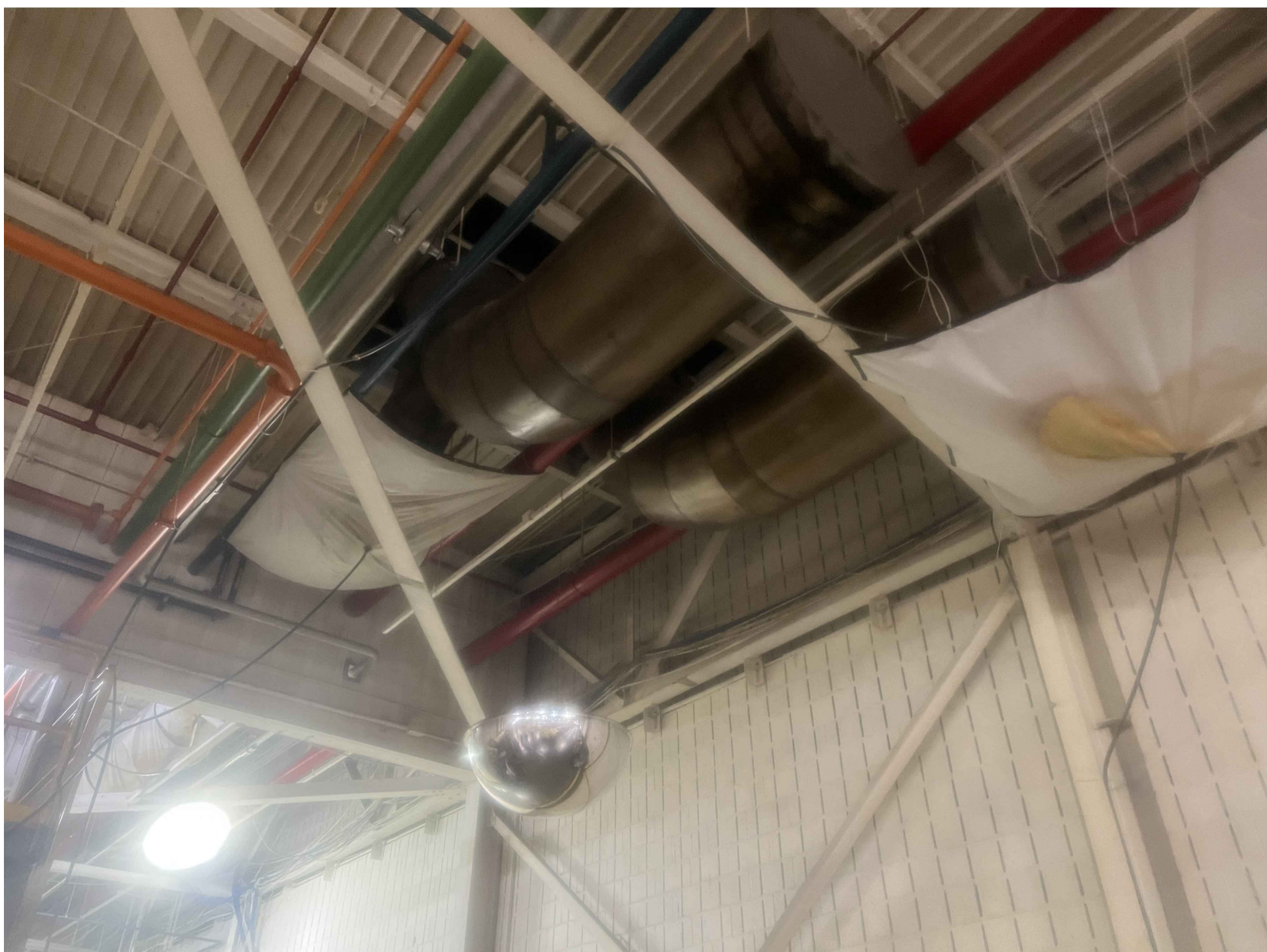
PHOTO No.04: EXISTING ABANDONED EXHAUST DUCTS
