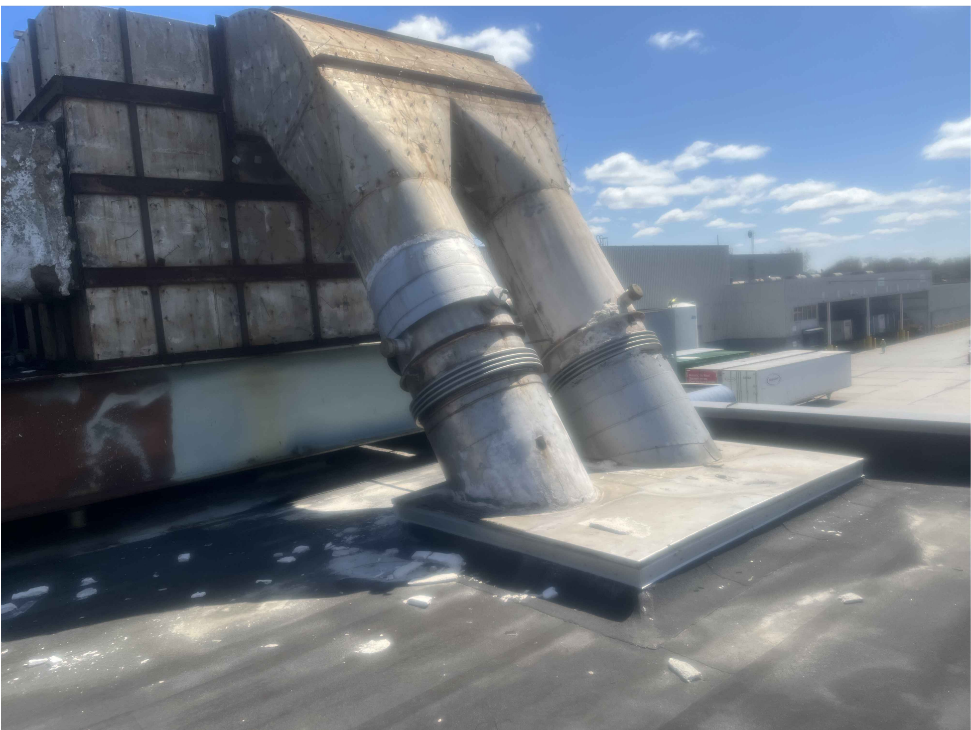
PHOTO No.06: EXISTING ABANDONED EXHAUST DUCTS
