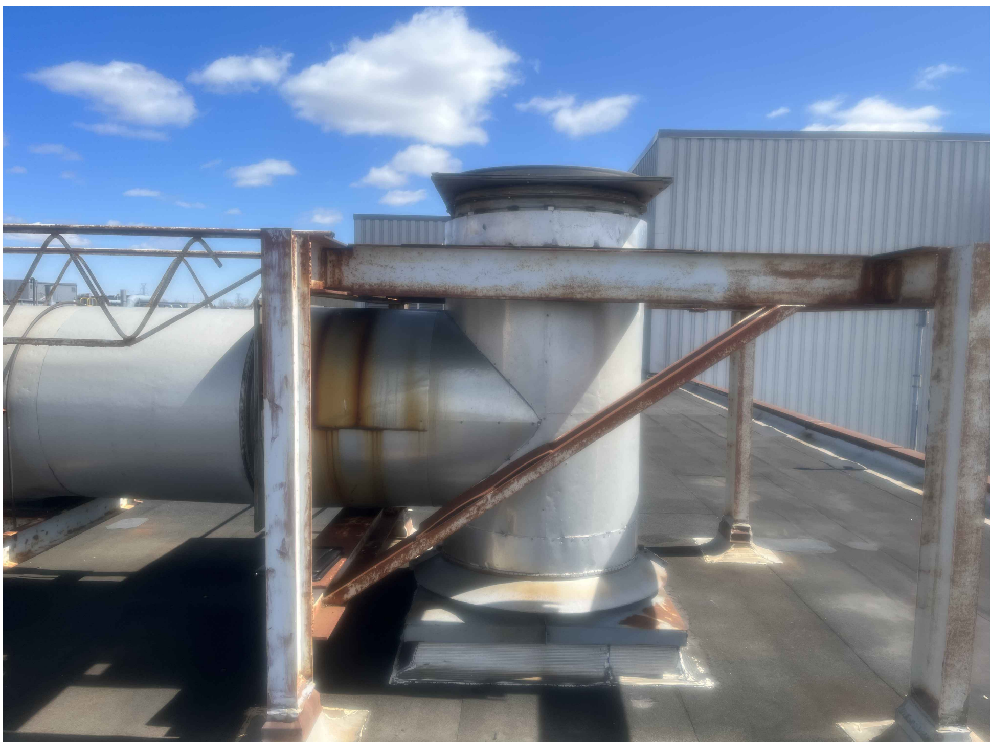
PHOTO No.07: TEST CELLS 101-114 EXISTING EXHAUST TEE
