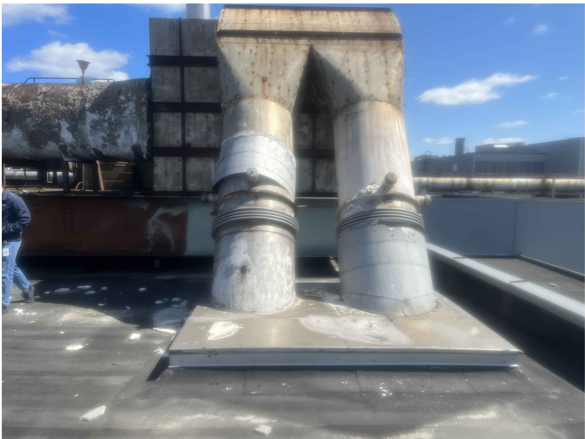
PHOTO No.05: EXISTING ABANDONED EXHAUST DUCTS
