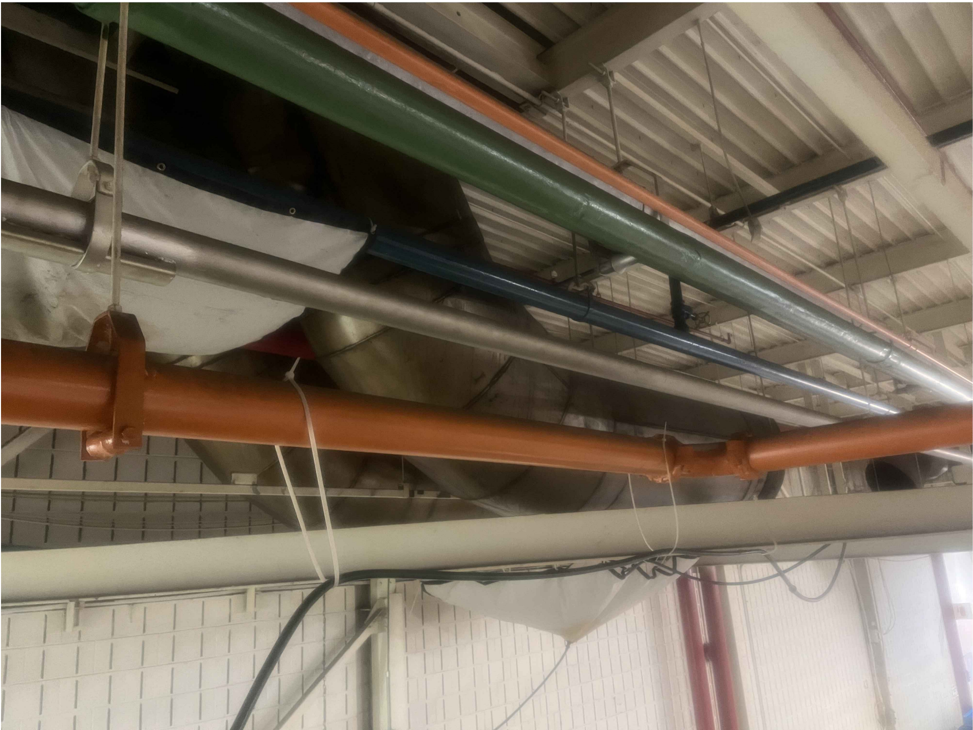
PHOTO No.03: EXISTING ABANDONED EXHAUST DUCTS
